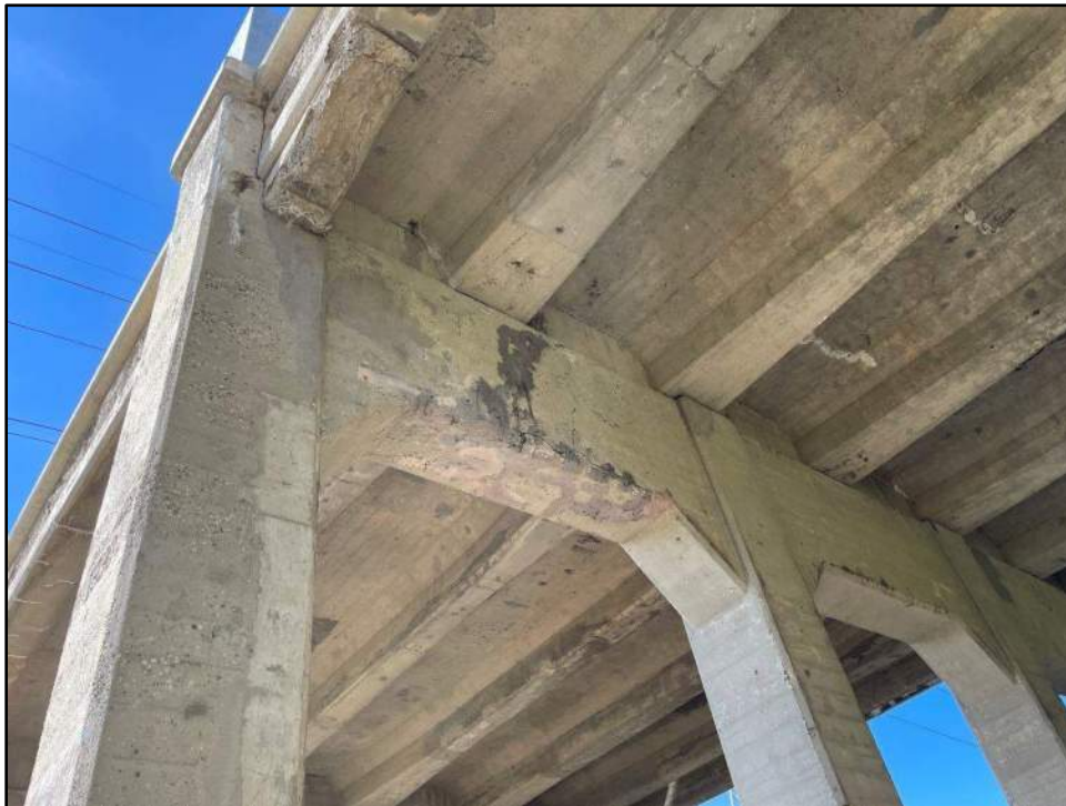
Previous deck and pier repairs near east pier
