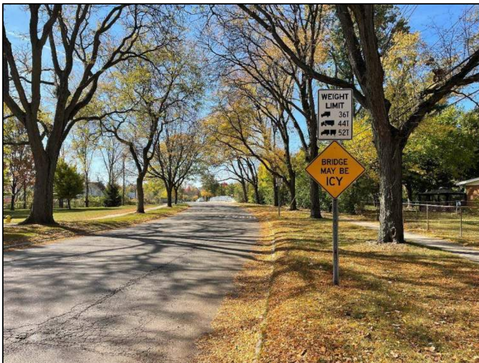
Approach looking southwest w/ posting sign (Old Posting)
