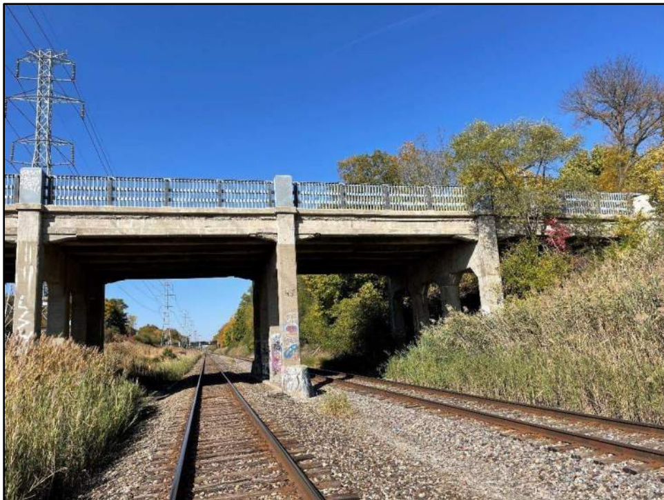
South elevation - east portion
