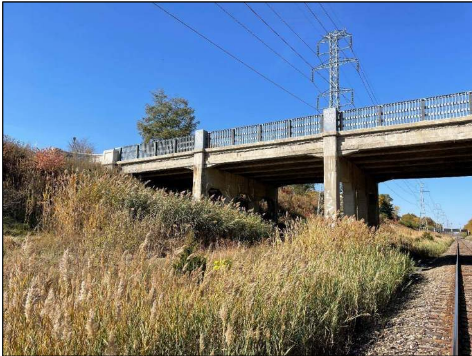
South elevation - west portion
